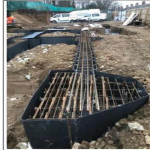
Description: Plot 53 – Block B Ground Beams
