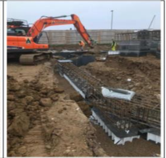
Description: Plot 53 – Block A Ground Beams
