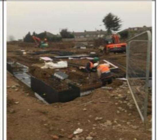
Description: Plot 53 – Ground beams
