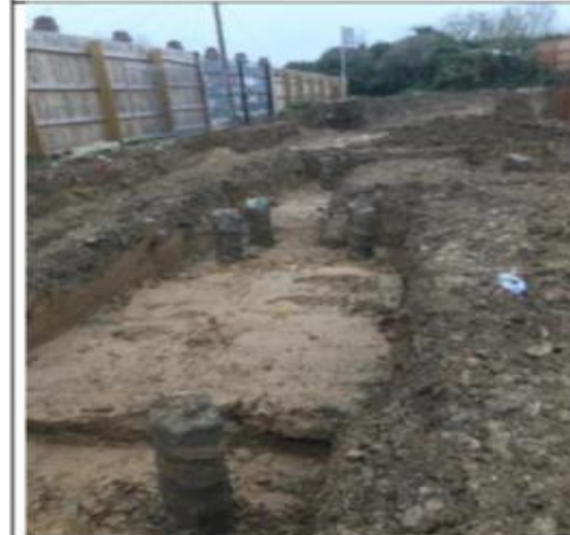
Description: Plot 54 – Block C Ground Beams
